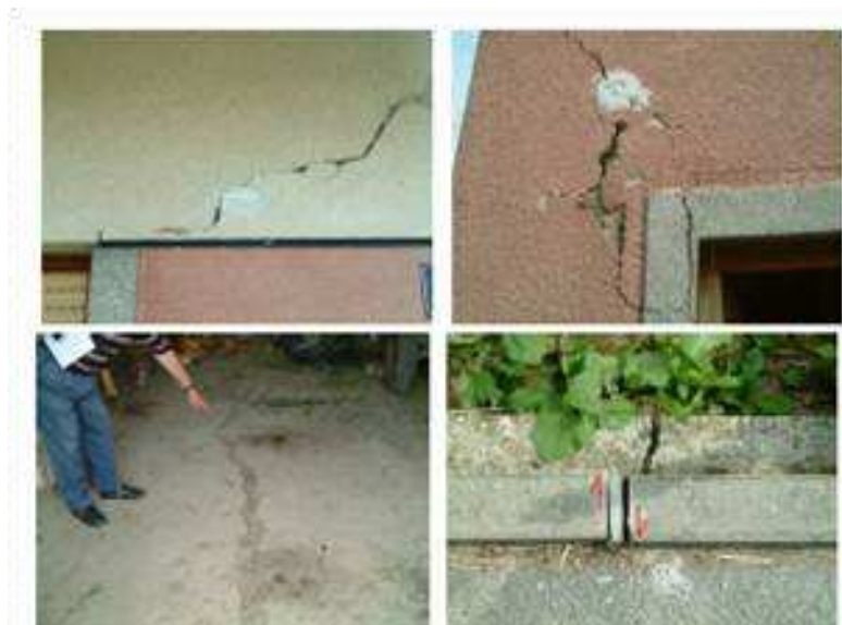
Figure 5 - Examples of damages on houses in the epicentral area near Zagreb.
