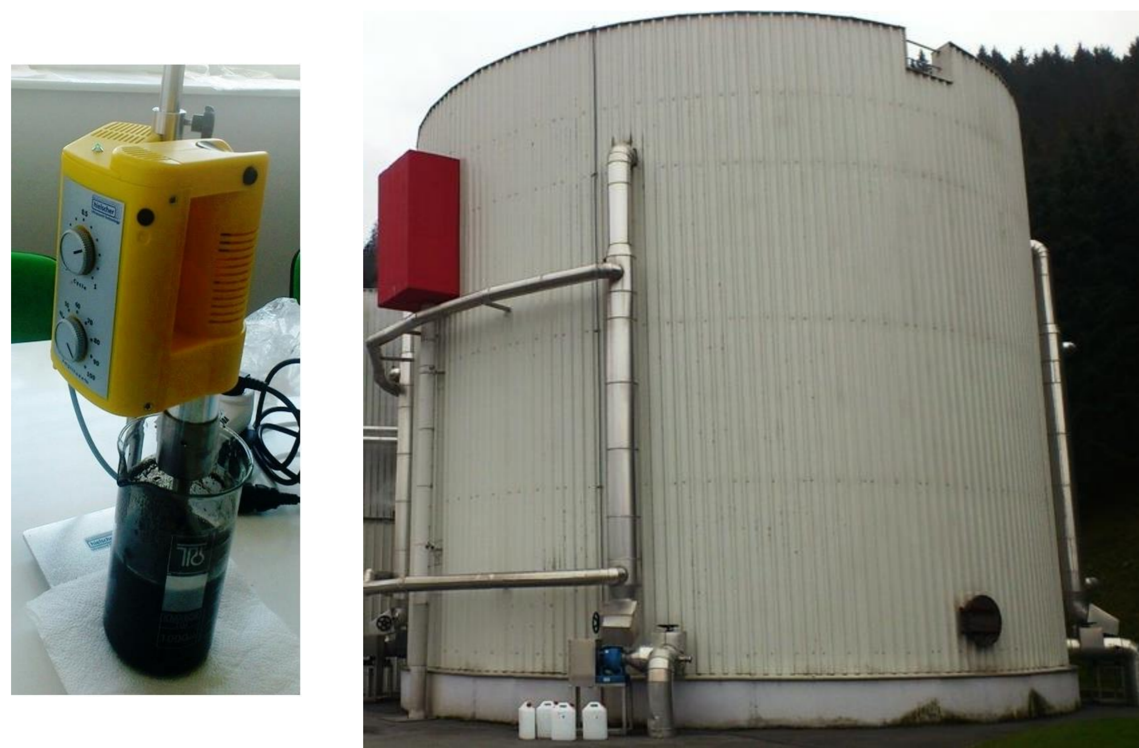
Figure 1: (left) Ultrasound homogenizator Hielscher used for pretreatment of wastewater sludge, (right) Anaerobic digester at WWTP Šaleška dolina.
